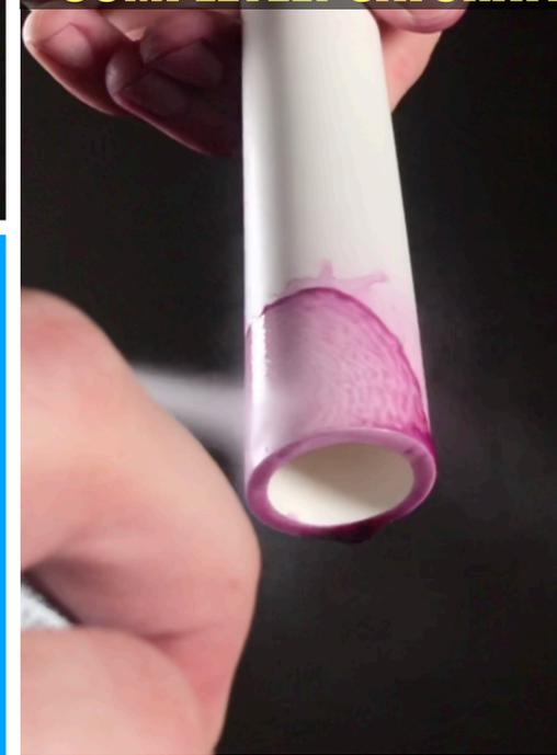
FOR A WATER AND PRESSURE TIGHT BOND, ENSURE THAT BOTH PIPE AND JOINT ARE SATURATED WITH PRODUCT BEFORE FITTING AND WAIT 60 FULL SECONDS BEFORE TESTING.
