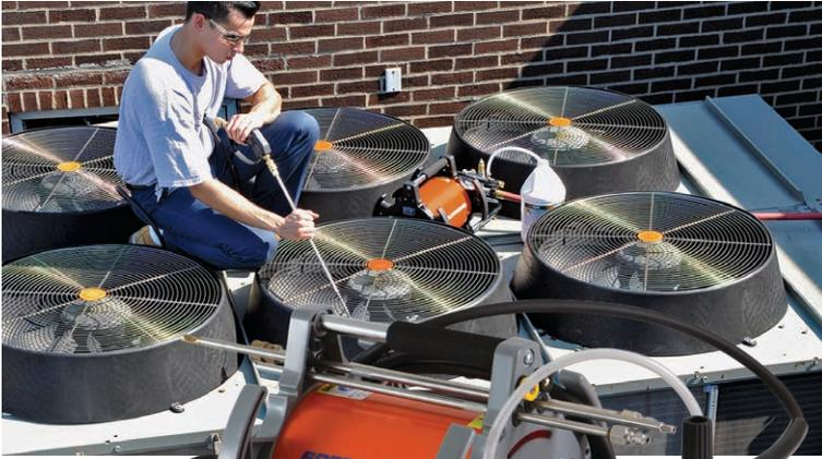
Water hose connection for continuous cleaning
