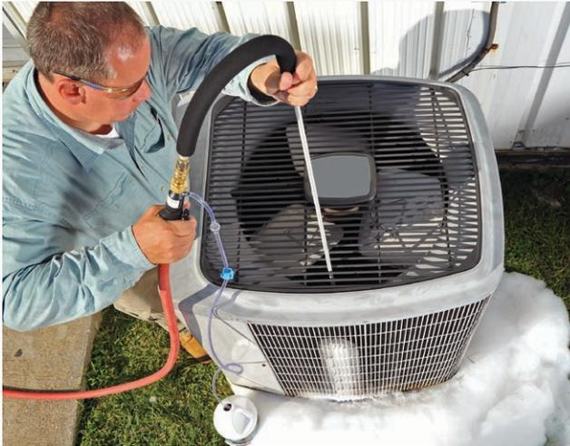
Swivel handle easily adjusts direction of water jet
