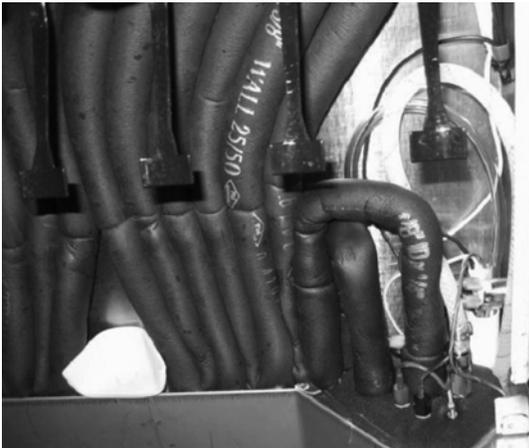
3. The carbonator tank purge tube (A) will be routed down through the valve leads conduit and out bottom of unit to a drain.
