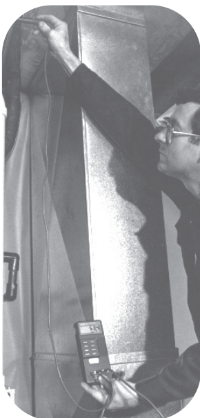
FIGURE 48 TEMPERATURE RISE MEASUREMENT
