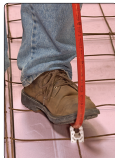
Protective plastic-to-plastic PEX connections
