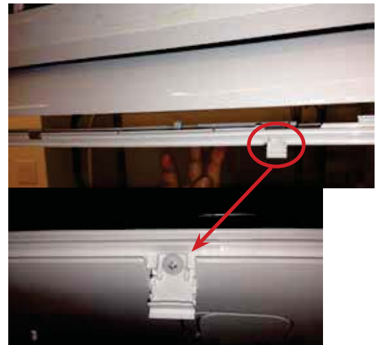
Figure 70: Latch over Screws on Indoor Unit Bottom Panel.
