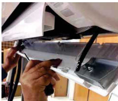
Figure 72: Remove Bottom Panel.
