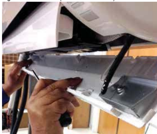
Figure 89: Remove (and Reattachment) Bottom Panel
