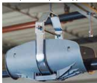
Examples of Piping Supports.
