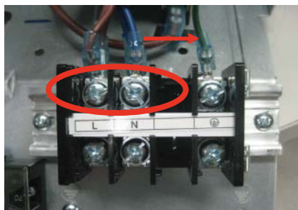
< Input Power Source Check Point >
