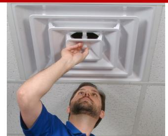
1. Easily attach to flex duct with cable tie/tape to pre-molded boot or boot added to Bulls Eye Back. Install Supply Back into drop ceiling grid without grille faces attached. Also available with Insulated Back option.
