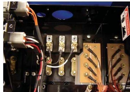
Figure 4.5 4D Voltage Sensor Connections
