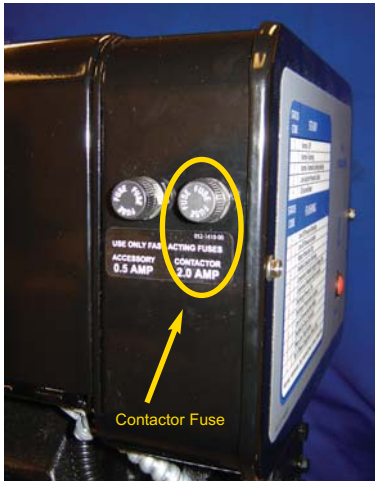
Figure 4.6 Contactor Fuse Location
